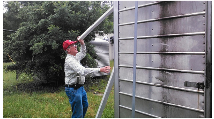
Pete adding wood, for the antennas to be off the roof for next time.
